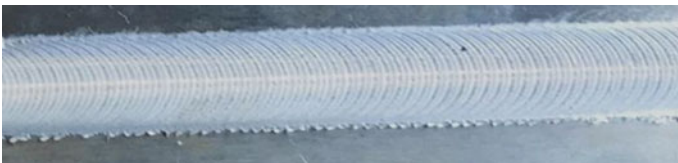
Fig. 7 Welded specimen surface of sample number 5. Smooth welded joint surface; no defects in welded joint (visual inspection); good welded penetration; no flash produced
